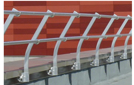
Figure 1 - Guardrail angled inward
